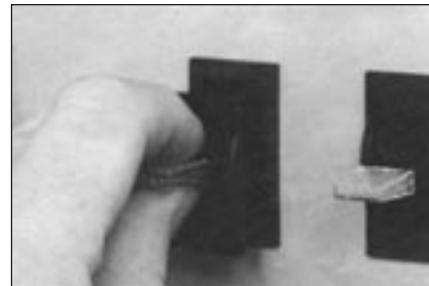
Replace lever assembly and "snap" escutcheon into place. Installation complete!
