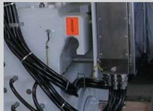
ring and insert are from PA6 (red for ISO metric and white for NPT).
