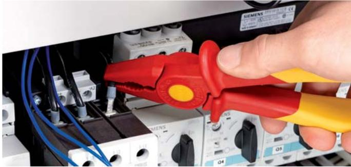
KNIPEX presents high-quality and sturdy plastic pliers featuring protection against bridging for working on live parts up to AC 1000V and DC 1500V.
