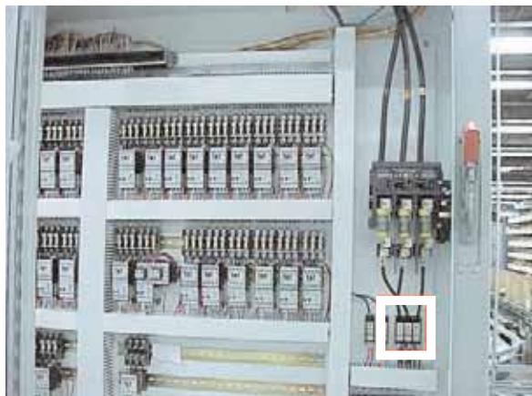
PDB in UL 508A, 480V Feeder Circuit must have spacing of 1" through air and 2" over surface. PDBs listed to UL 1953 meet these spacing requirements. Terminal Blocks recognized to UL1059 must be verified to have required spacing.
