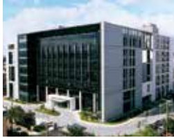
Taoyuan Technology Center (Green Building)
