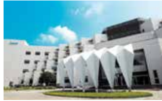
Tainan Plant (Diamond-rated Green Building)
