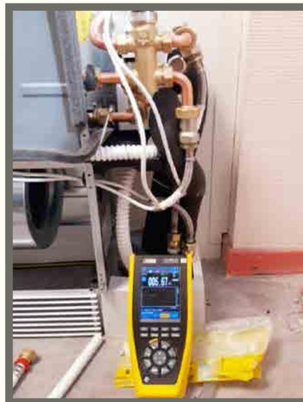
Measurements on heating and air-conditioning systems: current, voltage and temperature.
