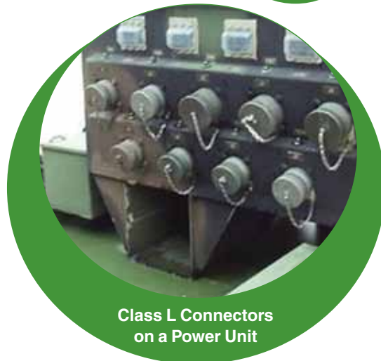
Class L Plug and Receptacle
